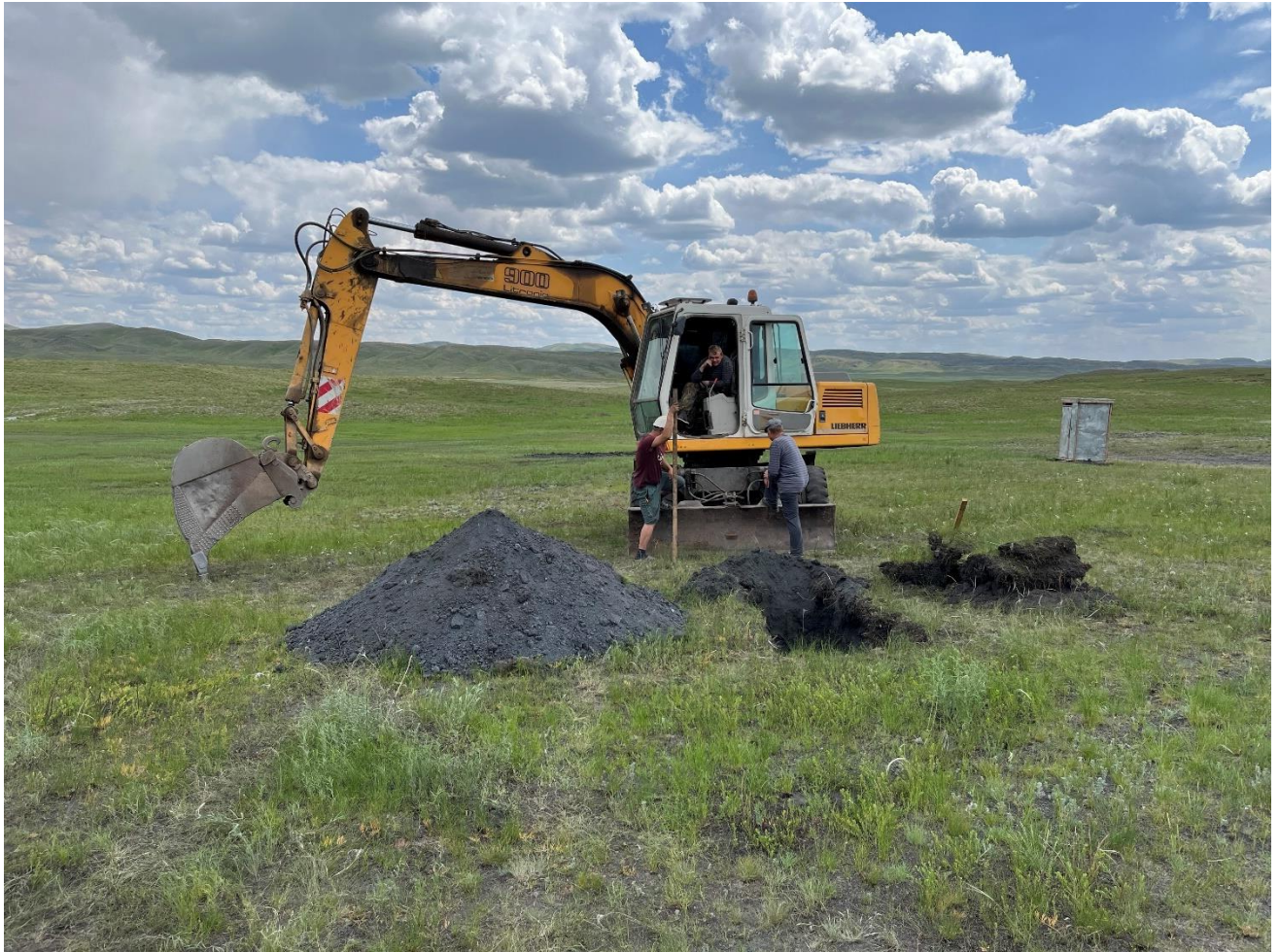
Figure 7 - Exploration test pit illustrating soft friable nature of the graphite mineralisation
